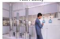
Automatic Helium Tightness Test Facility
