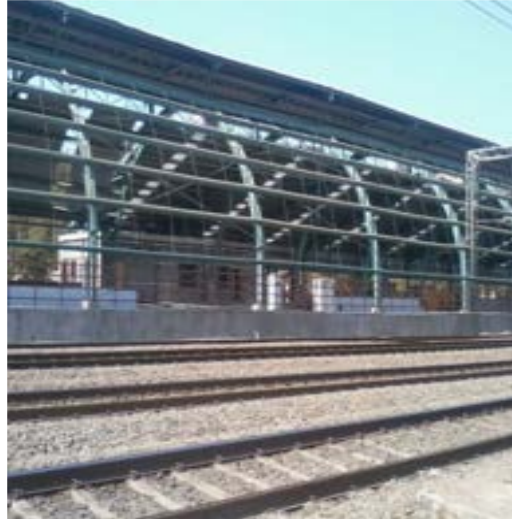
Construction of PEB Platform
