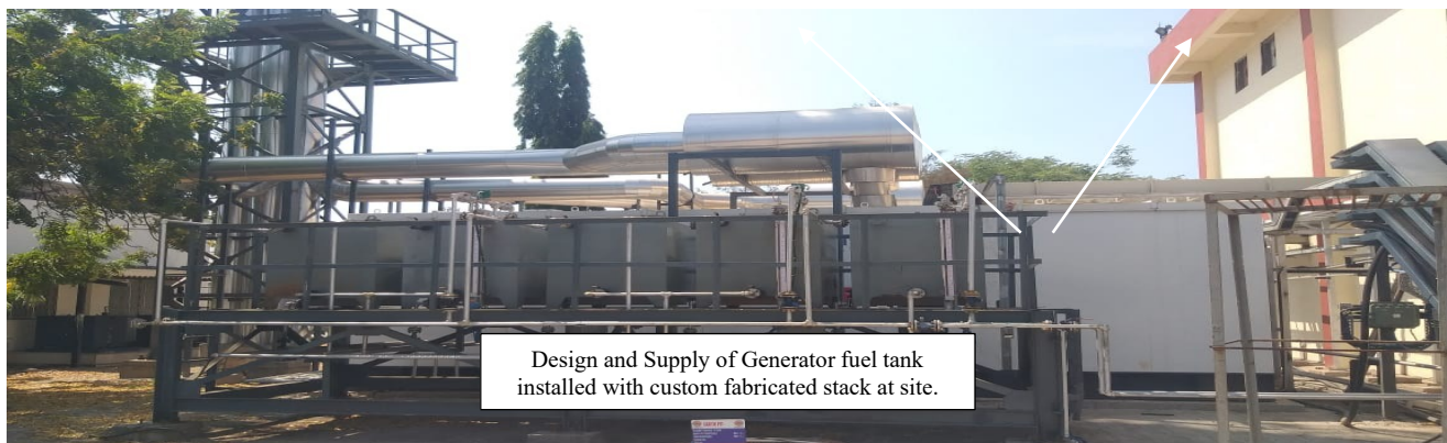
Fuel Tank for Generators
