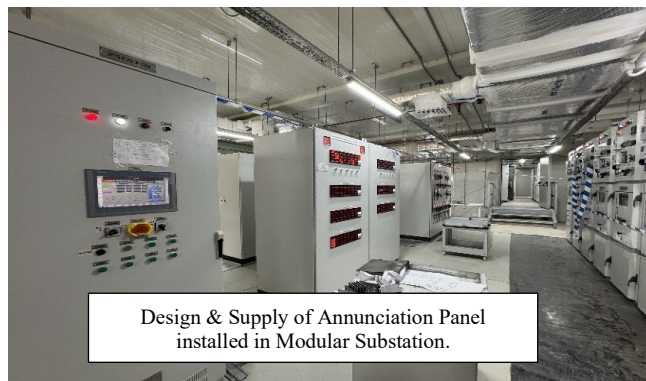
LV Panels and Annunciator Panels
