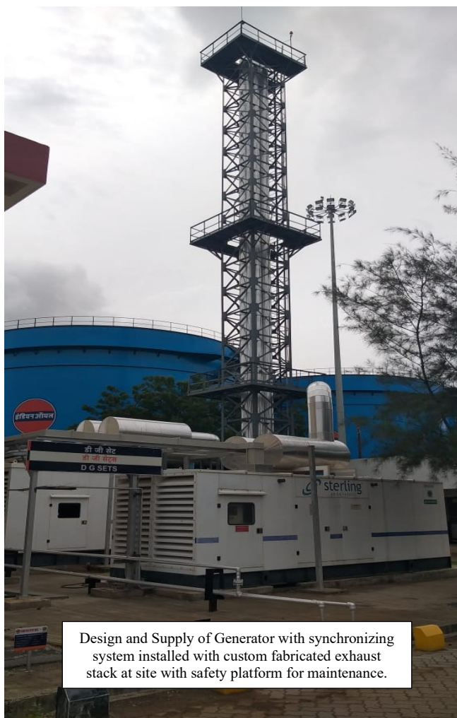
Generator with Exhaust Stack
