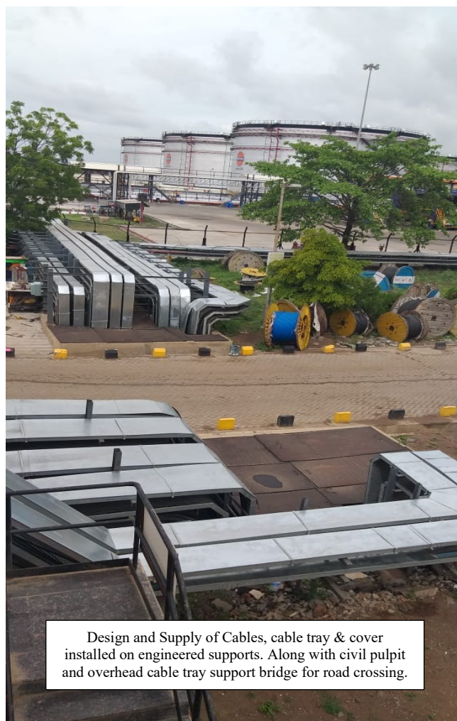
External Cabling System on Cable Trays
